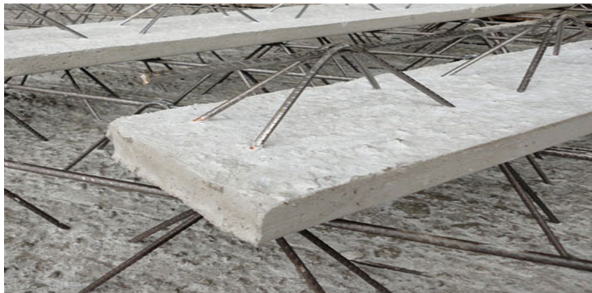
Finished rebar beam
